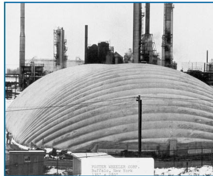
Figure 2, Exterior view of temporary dome sheltering entire work site
