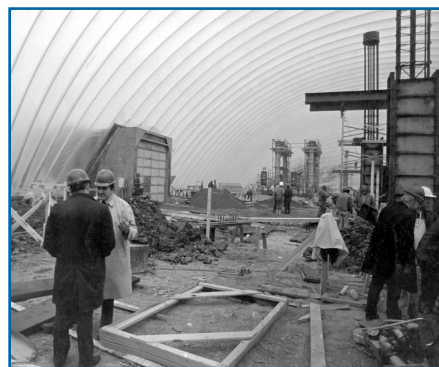
Figure 3, Dry, climate controlled, interior working environment.
